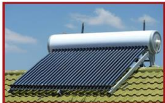
Solar Water Heater
